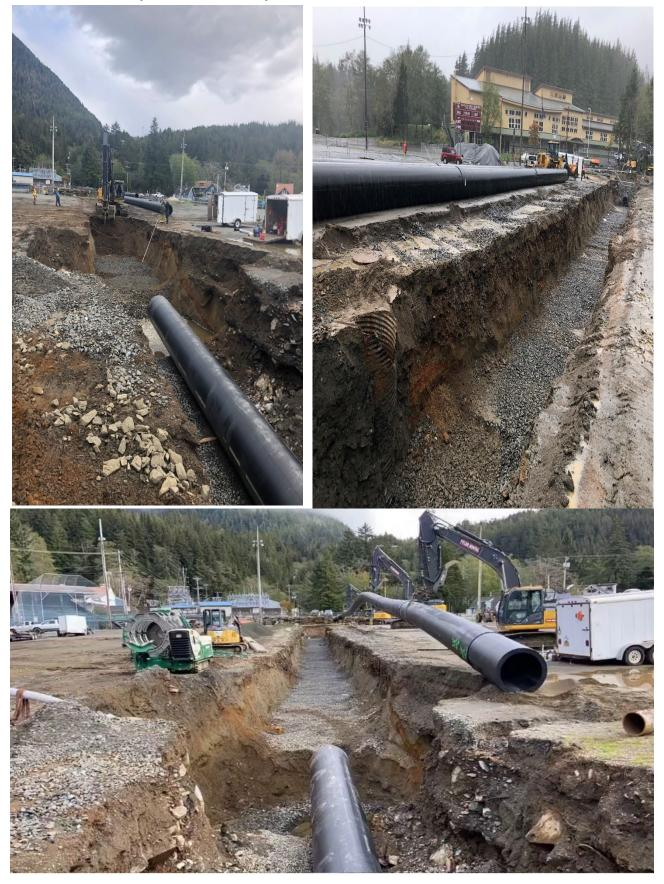
The last main-line segment was successfully lowered into the Walker Field trench by three hydraulic excavators on September 27<sup>th</sup>. By the end of October, this entire project should be substantially complete with the new 42-inch HDPE pipe segment installed and fully operational. The abandoned portion of the 36-inch ductile iron raw water main in Schoenbar Road will also be filled with grout to prevent future subsidence of the roadway.
