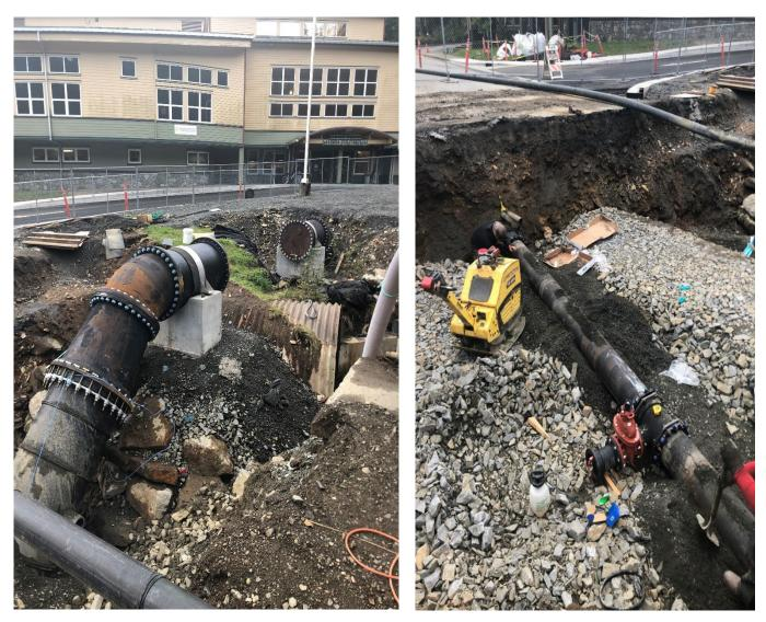
While Schoenbar Road was closed for the crossing, the existing 12-inch water main was intercepted and a 6-inch tee with valve installed for a future service to the planned Walker Field grandstands.
